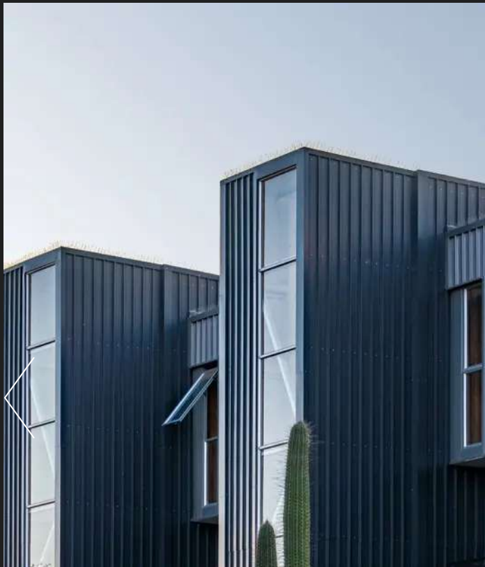
MODULAR CONCEPT IN AN ESSENTIAL SPACE. CONTAINER BUILDING BY HSU-RUDOLPHY ARCHITECTS
