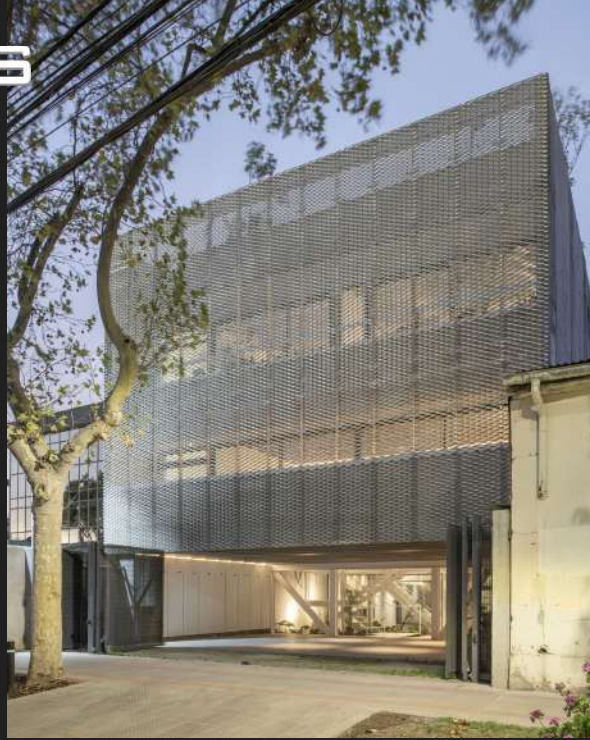
DSP apartment building in Santiago by Studio CL. Photograph by Bruno Giliberto.
