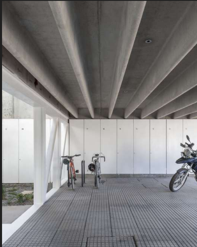
DSP apartment building in Santiago by Studio CL.
