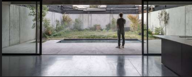
DSP apartment building in Santiago by Studio CL.
